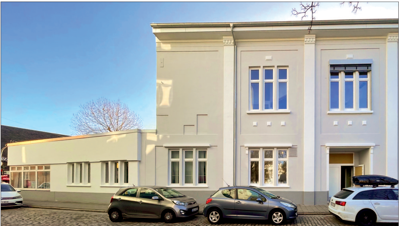
▲ The building of the planned "Arche" in Bremerhaven
